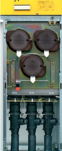
Raychem separable Screened Adaptors are designed to connect single-core polymeric cables to medium voltage equipment (transformers, switchgears, motors etc.) up to 24 kV.
