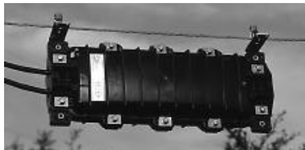
3M™ 2178-S case mounted on strand.
